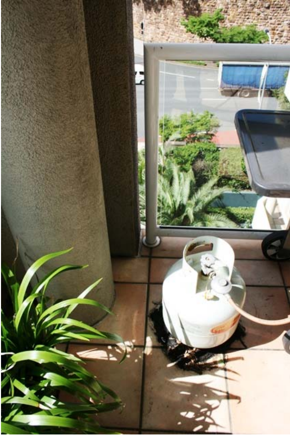
Photo 5 – Column to the balcony with glass balustrade.
