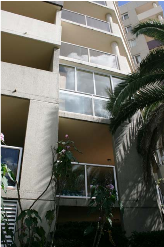
Photo 8 – Example of enclosed balcony with glass balustrade.
