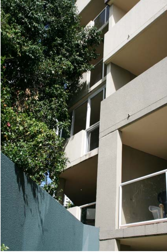
Photo 9 – Example of enclosed balcony with both a solid and glazed balcony.
