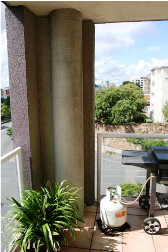
Photo 6 – Column to balcony with glass balustrade.
