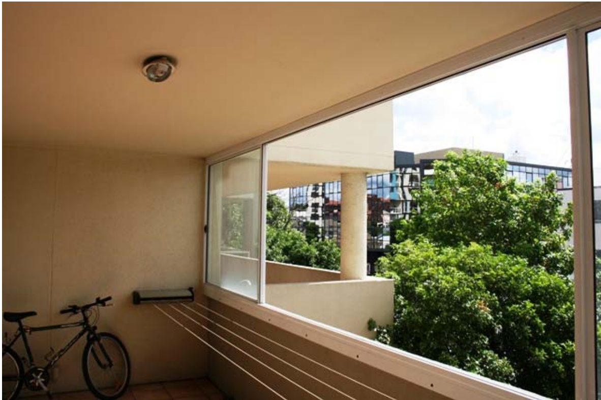
Photo 1 – Sliding windows to balcony with a solid balustrade from inside the apartment.
