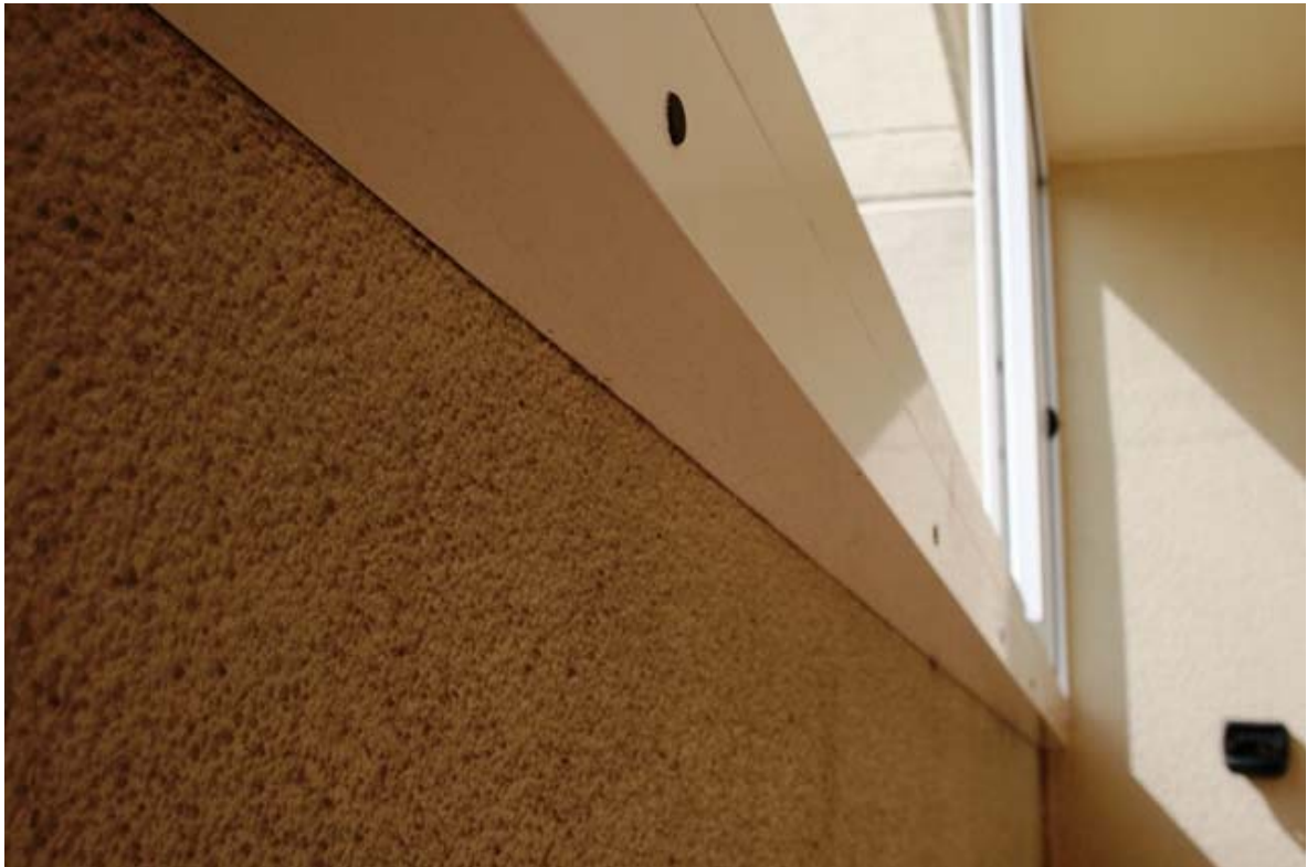
Photo 4 – Underside of sliding window sill track.
