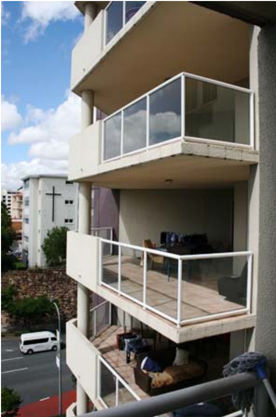
Photo 7 – Example of unenclosed balconies with a mix of solid and glazed balustrades.
